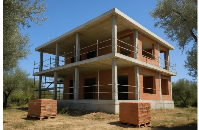
The shell structure seen from the lower side of the plot. Both slabs have been cast.
